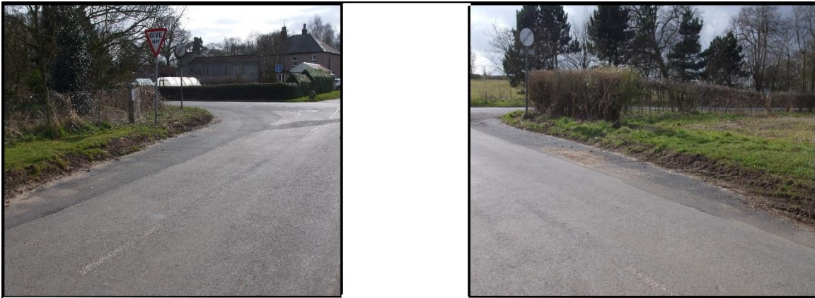
Photograph 3 Road Widening at Junction Smithfield Road and B1434
