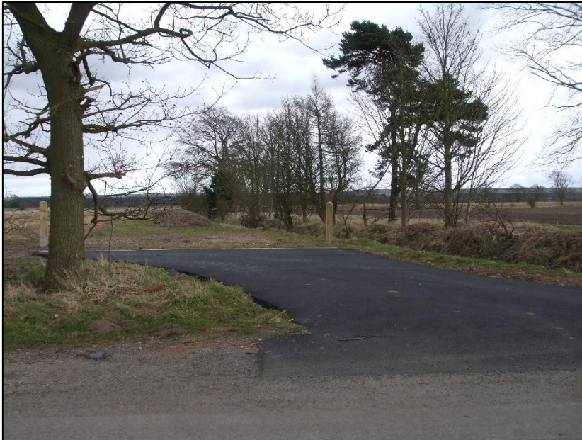
Photograph 1 Site Entrance as constructed 2018
